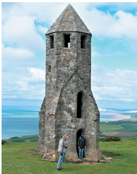
Fig. 1. St Catherine's Tower from the east, showing its upper and lower doorways and the peaked gable scar of its lost oratory. 2020
